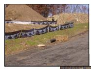
A simple tarp over this stock pile and geotextiles can help to avoid this problem.
