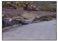
Exposed stock piles and soil can easily run off construction sites resulting in costly repairs clogging drainage structures.
